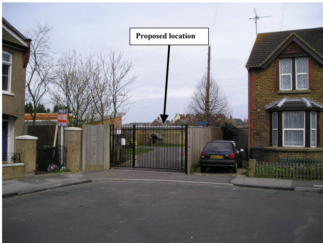
Photo 1 Pedestrian access from Arkley Road
